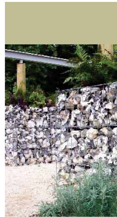
Flint gabion walls
