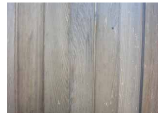
Cedar cladding to Hub
