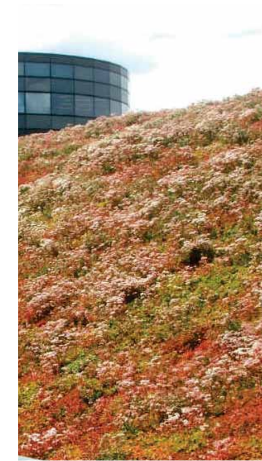
Hub sedum green roof
